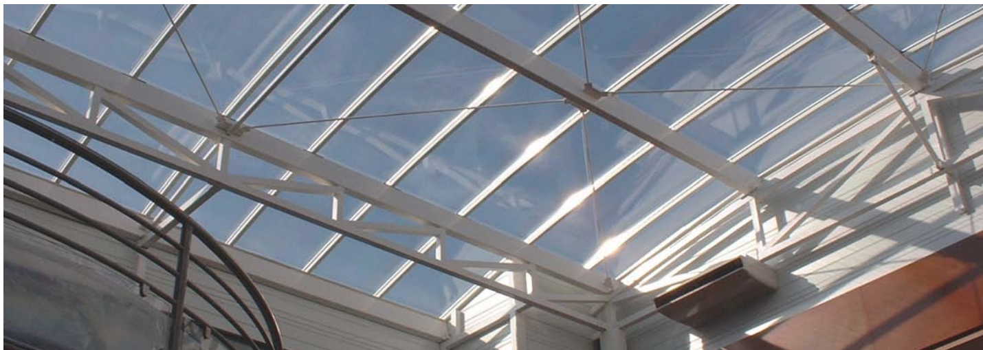
TPLV, Sandillon (45), Cabinet GAM architecture (75), sans lames brise-soleil
